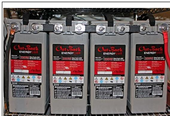
**Figure 6: String of four AGM batteries**
