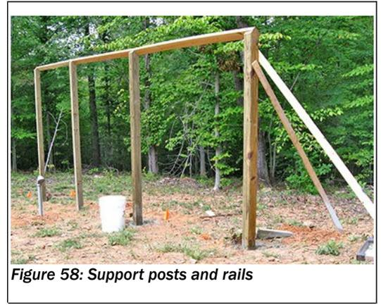
Figure 58: Support posts and rails
