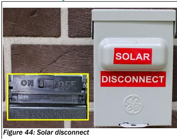
Figure 44: Solar disconnect
