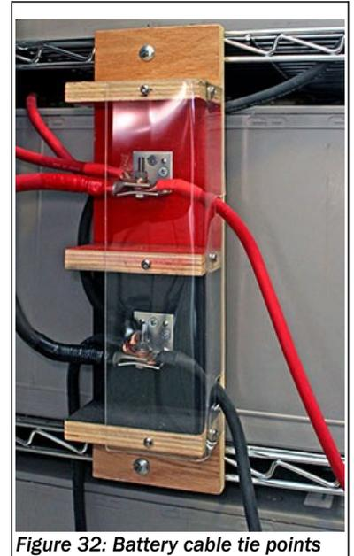
Figure 32: Battery cable tie points
