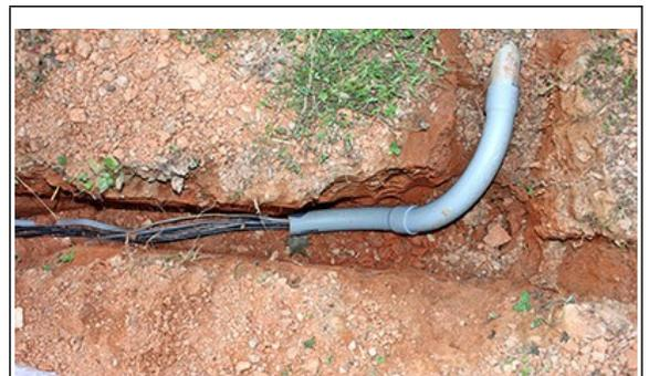
Figure 42: Feed cable conduit into house
